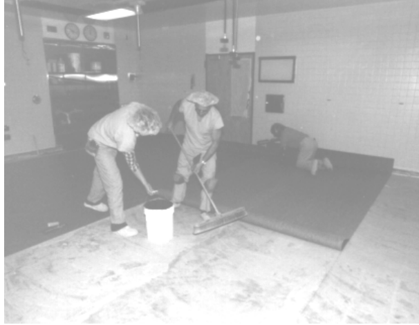
Fig. 3.4.2.1 Lav Out Oversize Sheets And Broom Clean
