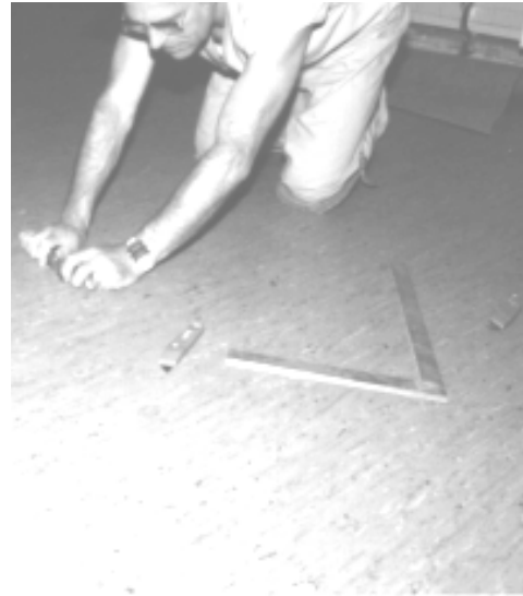
Fig. 3.4.2.3 Feathering All Areas Manually With A Cork Smoother: This prevents entrapped air from forming bubbles and hollow spots.
