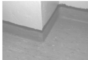
Fig. 3.6.2. Hot air Puttied Inside/Outside Corners over Patch Levelled Wall.
