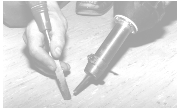
Fig. 8.1. Diagonally Cut Perimeter of Damaged section Section
