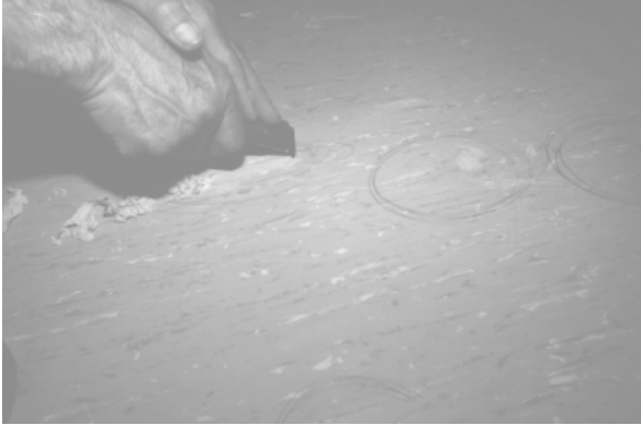
Fig. 8.7. Repairing of a Burn
