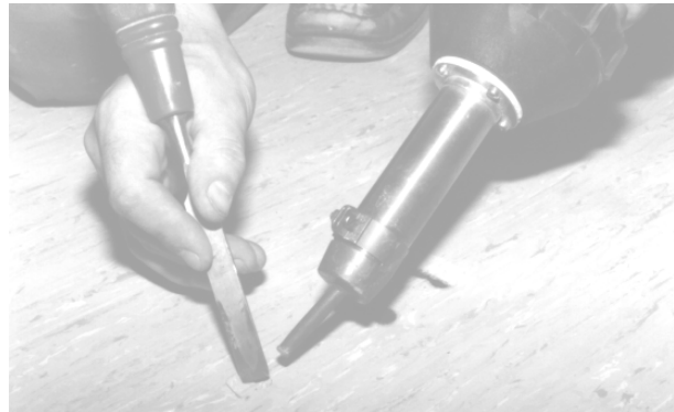
Fig. 8.3. Using Roller to Insert Repair Piece
