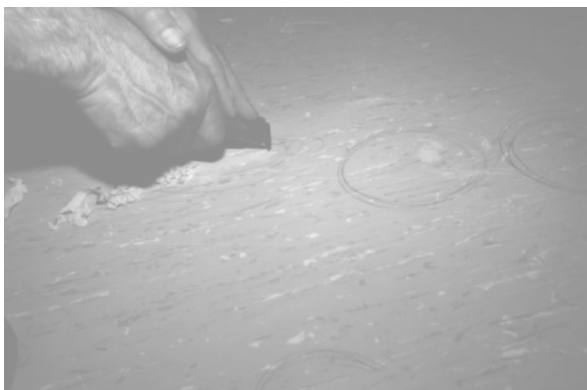
Fig. 8.7. Repairing of a Burn
