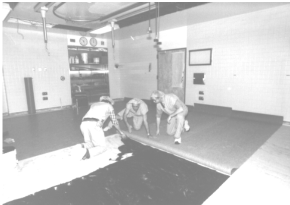
Fig. 3.4.2.2 Folding Back Vinyl and Troweling Approx. 200 sft. (shown with a black Conductive Adhesive not TSC-100 adhesive)
