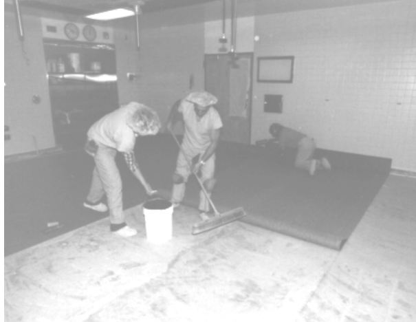
Fig. 3.4.2.1 Lav Out Oversize Sheets And Broom Clean
